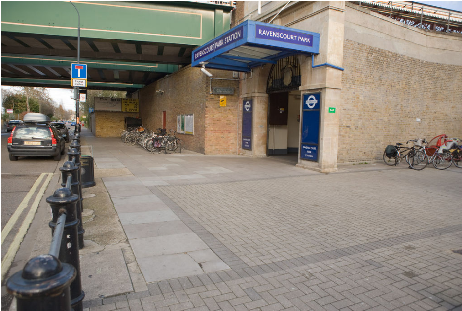
Footway outside station entrance
